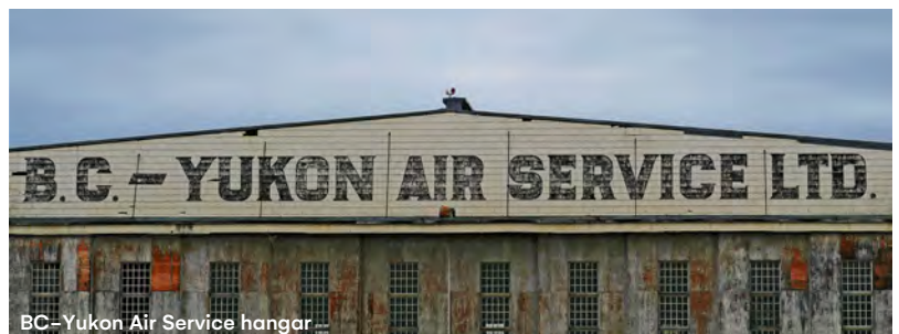
BC-Yukon Air Service hangar
